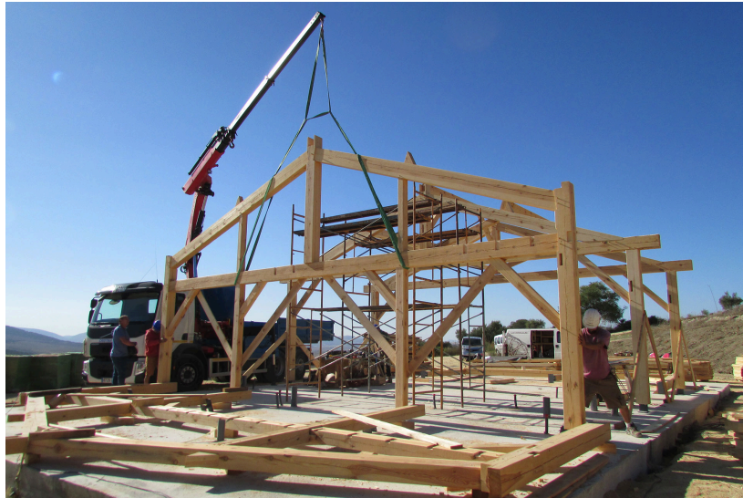
Figure 8. Learning Wooden structures carpentry at the building site. Author: Loris Carboni
